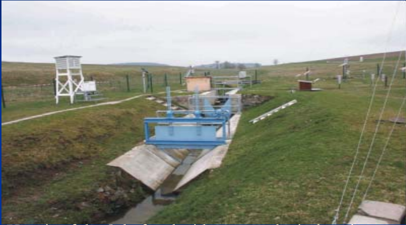
V-weir of the Schäfertal with meteorological station.
